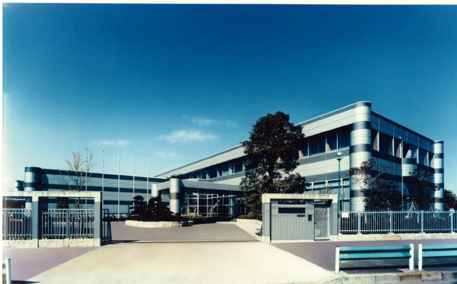
Fig.3. The new SRL building in1988.
